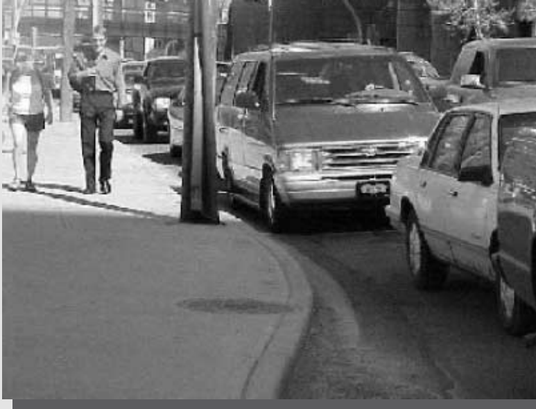
Exhibit 5. Local deficiency associated with narrow curb lane width on 6th Avenue S.W. at Centre Street, leaving very little space for motorists to overtake cyclists.
