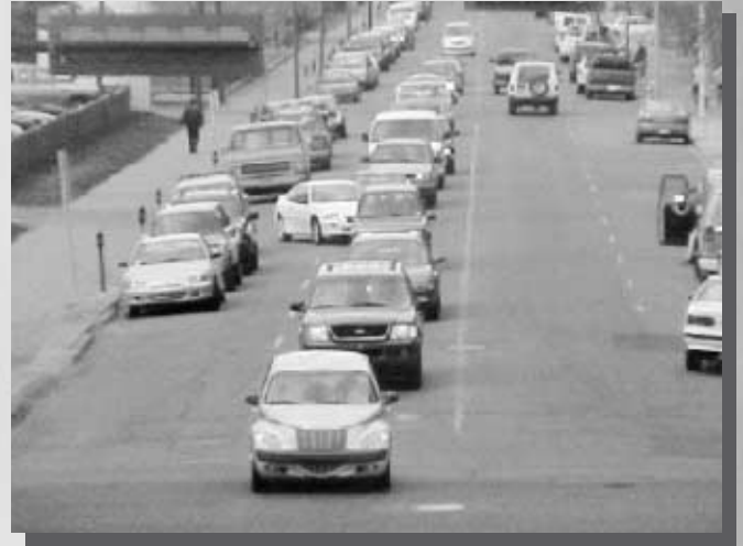
▲ Exhibit 2. Typical on-street environment in Downtown Calgary. Note how part of the parking lane might be used by the cyclist, yet might also present hazards such as opening car doors and cars accessing the roadway.
